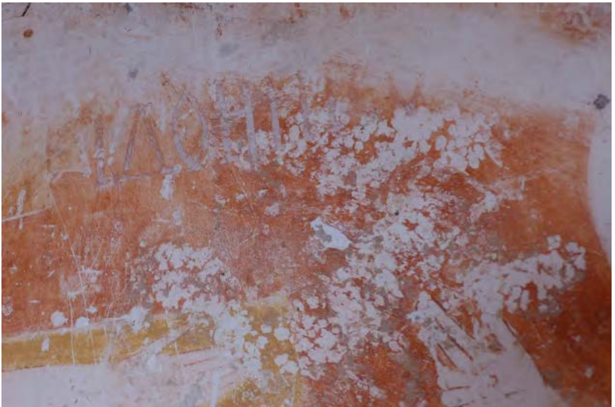
Figure 33. Remains of earthen nest material, and loss of the paint layer where it has been removed
