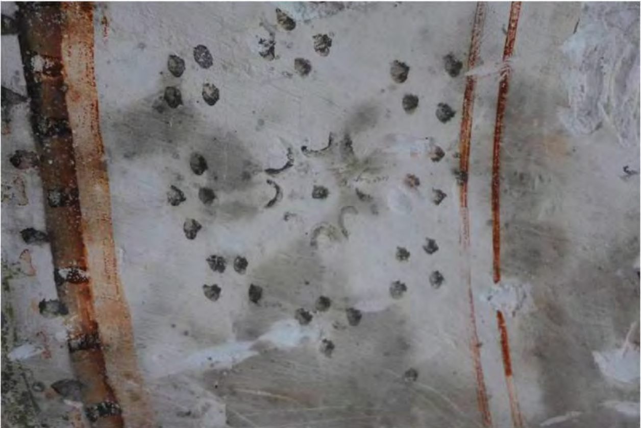
Figure 34. Grey veil which seems to be of biological origin
