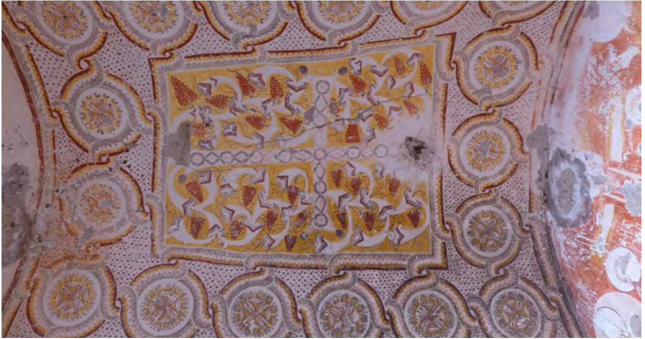
Figure 14. A structural crack can be seen running through the plaster and paint layers on the ceiling of Chamber 2, from east to west
