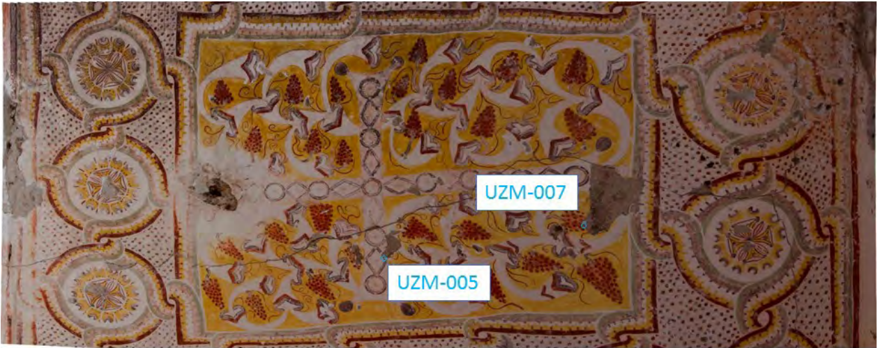
Figure 8. Paint sample location in Chamber 2, ceiling.
