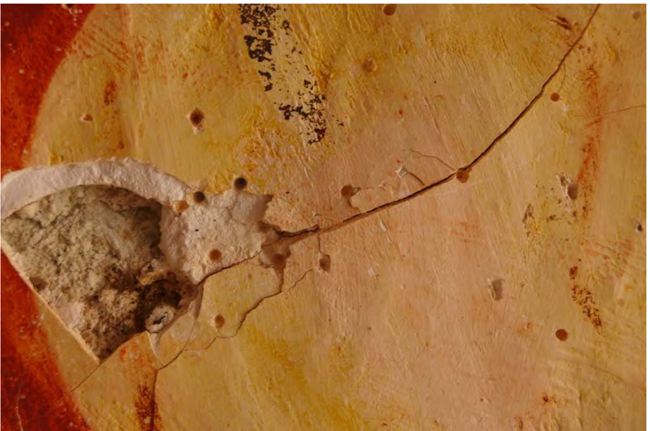
Figure 26. Small and homogenous holes were observed in the plaster layer. Their origin is unknown
