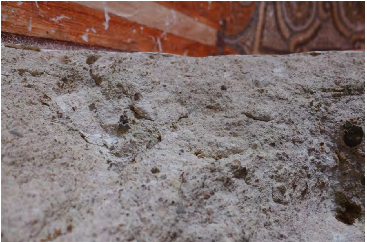
Figure 15. Spalling of the stone was observed in some areas
