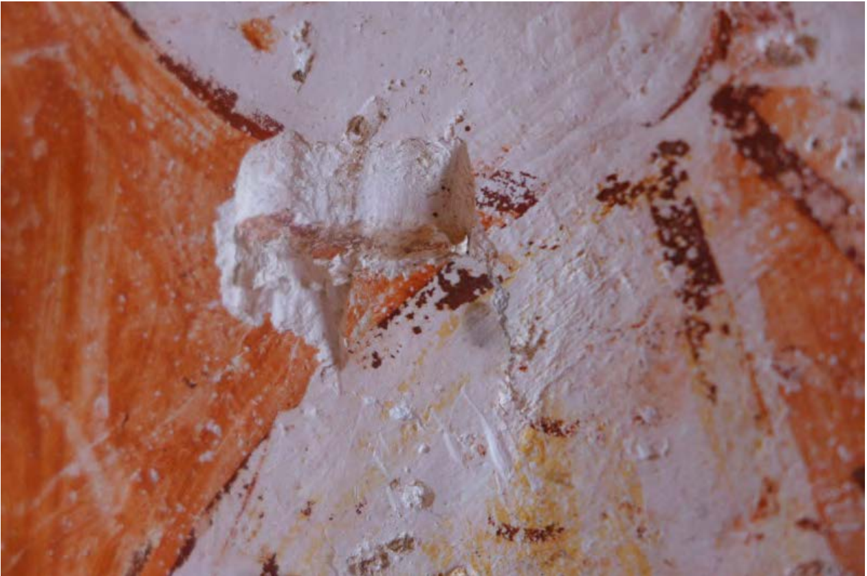
Figure 8. Where damaged through impact, the plaster appears fractured but compressed, suggesting that it is quite a soft material
